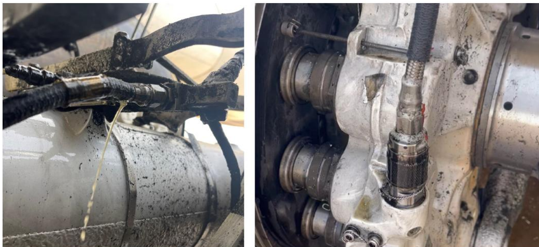
Figure 12 Blue Hydraulic brake lines leak.
