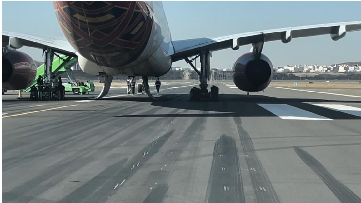
Figure 14 Runway 18 light surface depth “white color scar” damage.
