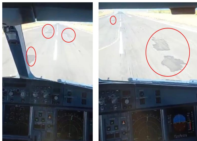
Figure 28 Photo showing the condition Comoros runway on the day following the event
