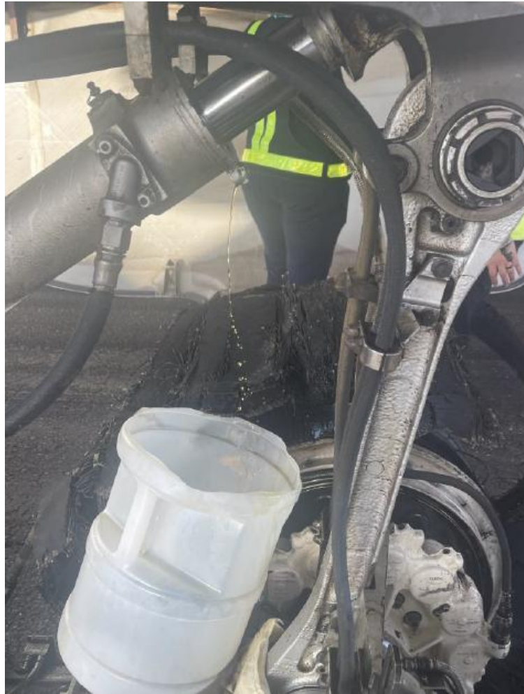
Figure 9 The right trimmer actuator was leaking.
